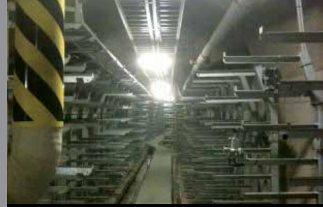
Prague City Utility Tunnels, Czech Republic
