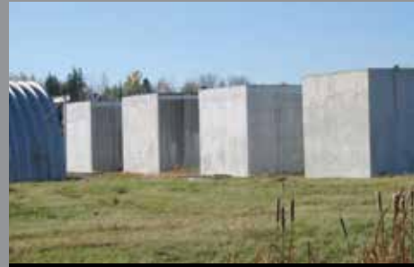
Nuclear Waste Storage Bunkers, Canada
