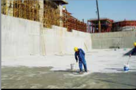
Coal Storage at Power Station, China
